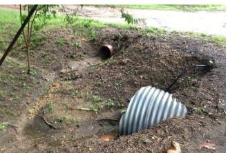
Figure 7A: Damaged Culvert Example
