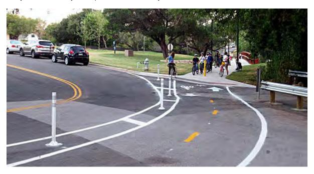
A protected bike lane provides a connection to an existing sidewalk in Austin, TX<sup>88</sup>
